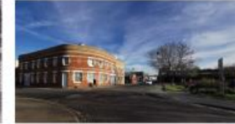
Fascadism of newly converted Great Eastern Road corner block
